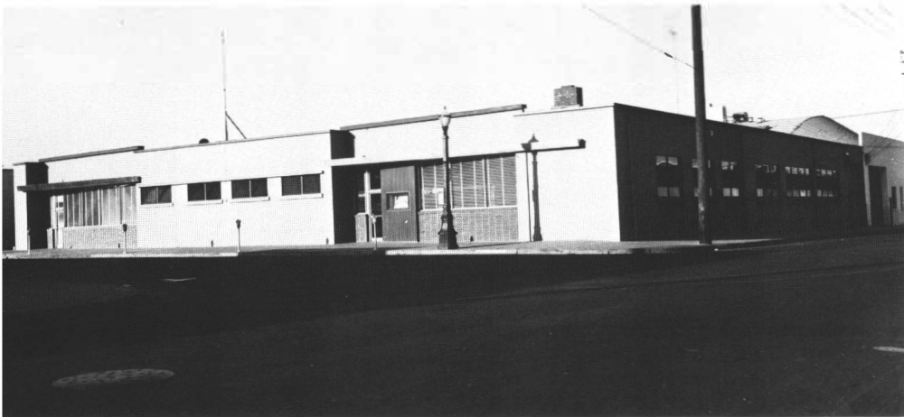
The original building that housed the IBM Research and Development Laboratory. The first unit, on the corner, was 10,000 square feet in 1952, and was enlarged to about 18,000 square feet in 1953.
