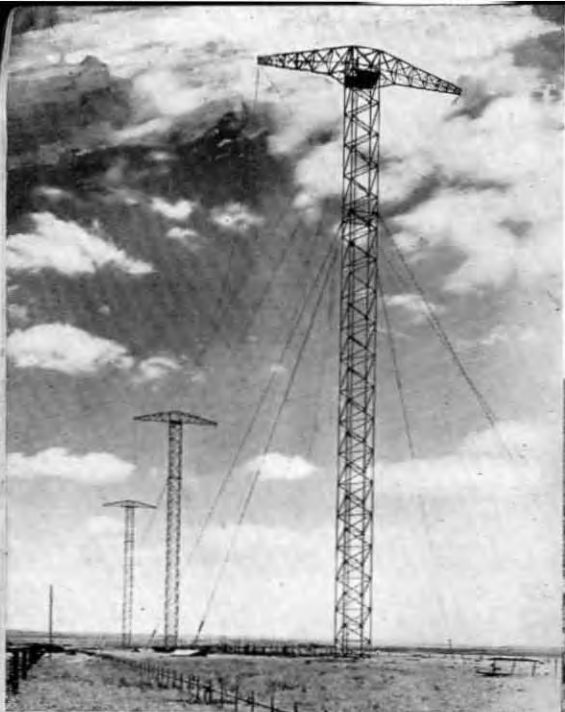
Beam Aerial Masts, at Fiskville, Victoria
