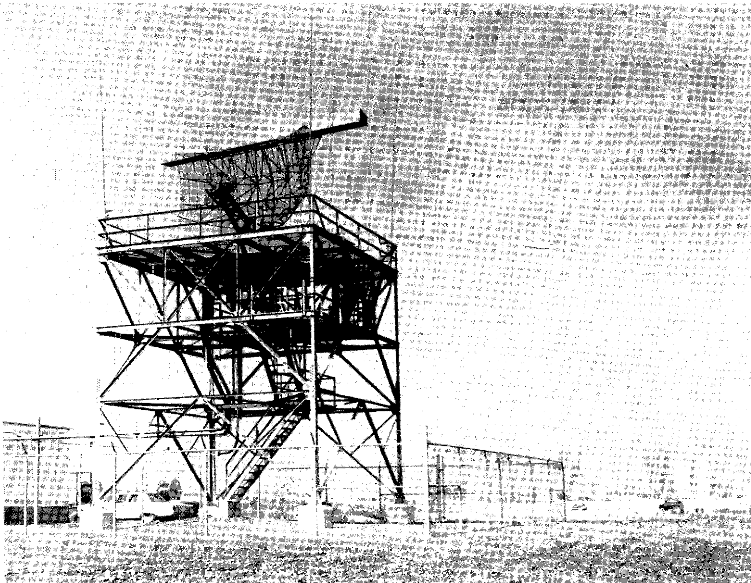
Fig. 14. ATCRBS hogtrough installed on ASR reflector.
