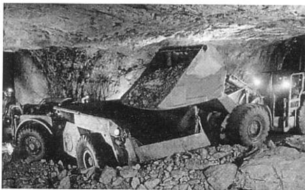
Loading and hauling ore at the Friedensville Mine, ca. 1976. (Courtesy of Ken Cox.)
