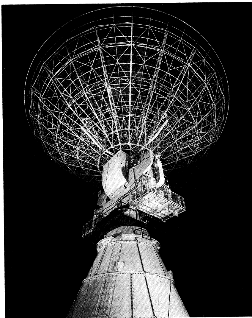
Figure 14. AN/FPS -49 BMEWS search-track radar (photo courtesy of RCA).
